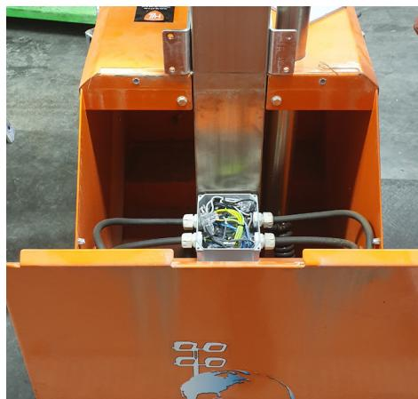
2. Open the terminal box and disconnect all the cables that run to the ballasts. Connect the incoming cable with the outgoing spiral cable that runs up inside the mast, either inside the terminal box or using a quick connector (earth, phase and neutral conductors that run up mast).
