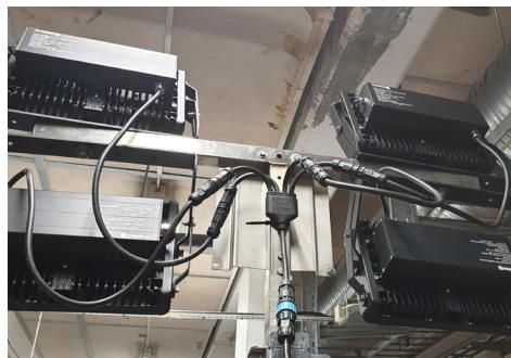
6. Secure the spiral cable to the plate on the crossbar using a screw.
